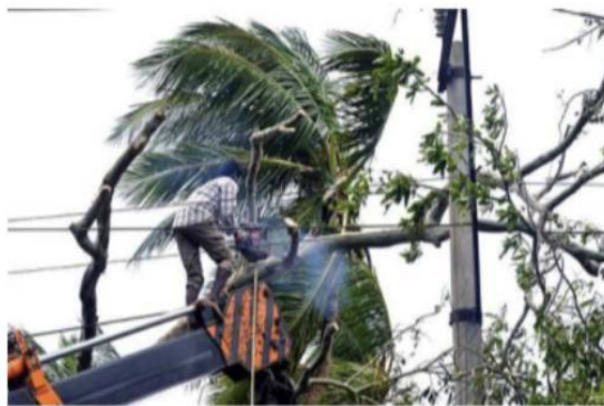
Power restoration work in progress near Bendamurlanka in Dr. B.R. Ambedkar Konaseema district on Wednesday after Cyclone Arnab makes a landfall. V. RAJU
